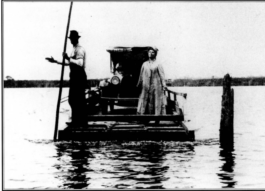
Going to Florida, on St. Mary's River, Georgia, 1917
